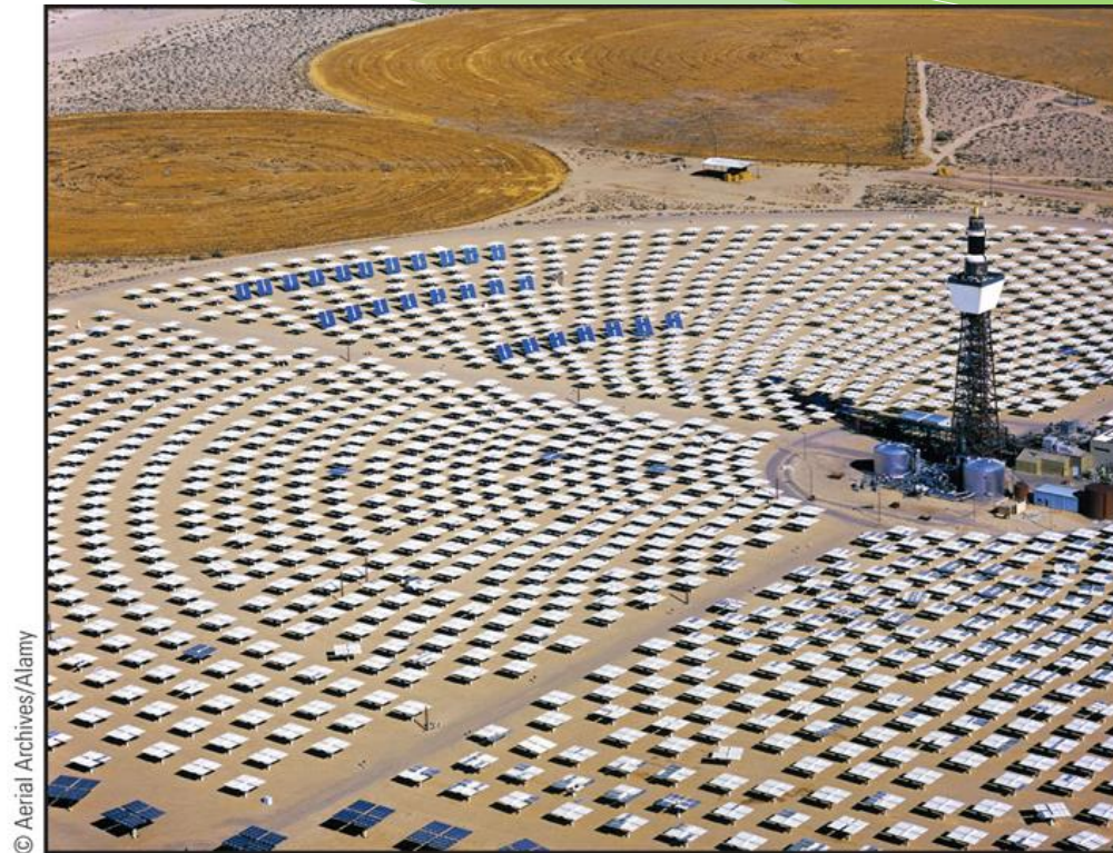
Figure 9.4: Solar Two in Daggett, California. The scale can be determined from the central tower that is about 90 m high.
