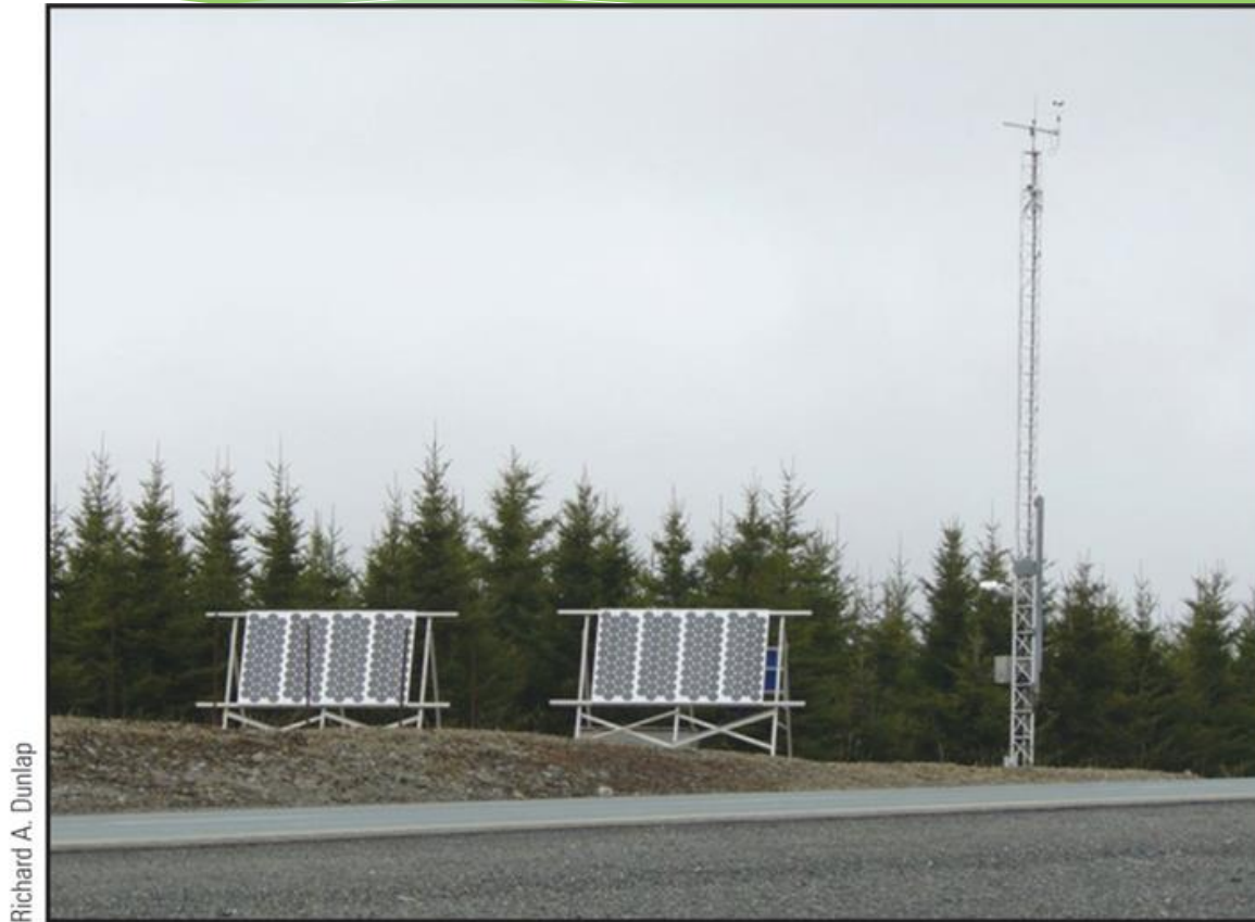
Figure 9.25: Photovoltaic array for providing power at a remote radio transmitter station.
