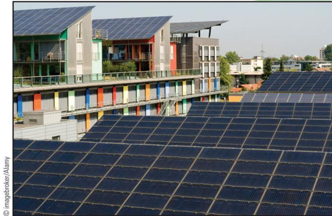
Figure 9.26: Photovoltaic solar panels on homes in the Solar Settlement in Freiberg, Germany.
