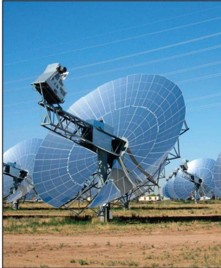
Figure 9.3 Parabolic dish solar collectors at Maricopa Solar Project in Peoria, Arizona showing the Stirling engine used to convert heat to mechanical energy.
