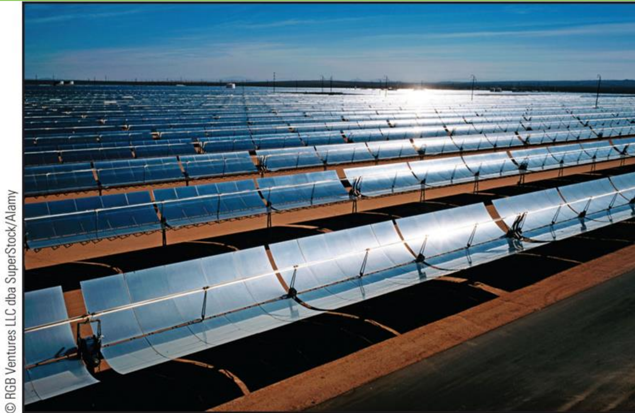
Figure 9.1: Parabolic trough solar collectors at Kramer Junction, California.
