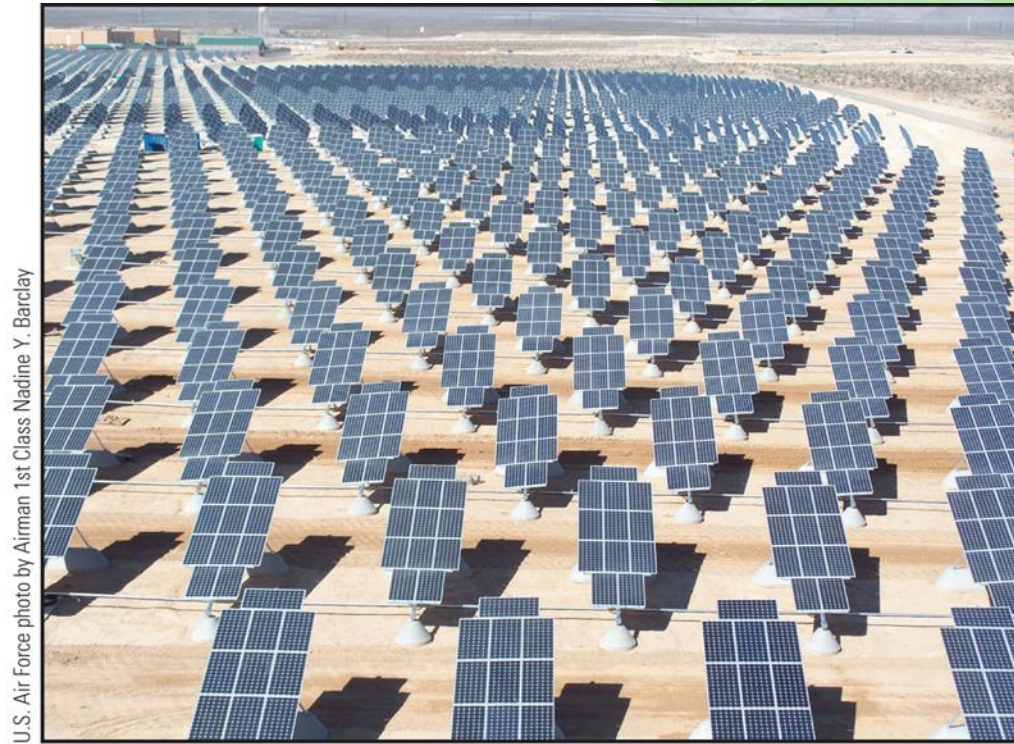
Figure 9.30: Photovoltaic arrays at Nellis Air Force Base, Nevada.
